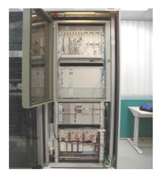
A redundant gateway CPC with the WIN-NT4.0 operating system couples the decentralised RFC of the pre-cut conveyor line with the AC450 Advant controller. The OPC server of that gateway communicates with the decentralised RFC clients of the drive stations and the OPC client of the CI546 TCP/IP interface in the AC450.
